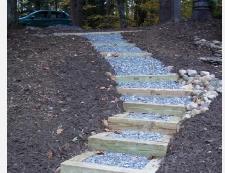
Infiltration steps protect steep slopes w/foot traffic
