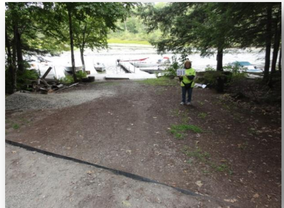
A rubber-razor needs repair to hold back soil at this commercial camp in Sector 2.
