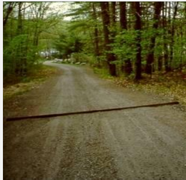
Rubber razors direct water off driveways and into vegetation
