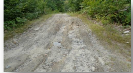
An eroding private road site on Homestead Rd. in Sector 1. New surface material, runoff diversifiers and ditches are needed.
