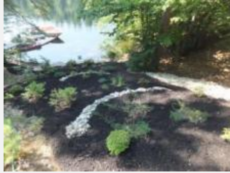
Erosion control mulch & vegetative planting
