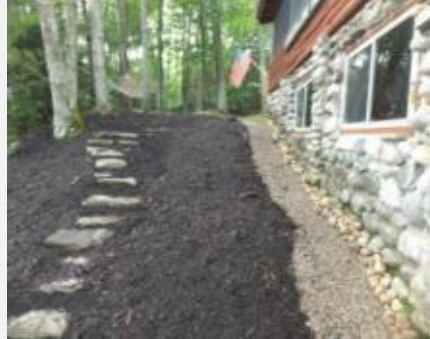
Dripline trench & erosion control mulch (Photo: AWWA)
