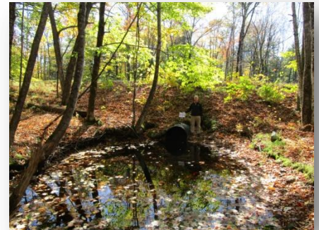
A large scour pool at the outlet of the Castle Island culvert in Sector 16.
