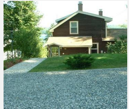
Resurfacing driveways with hard-packing, cohesive surface material prevents erosion
