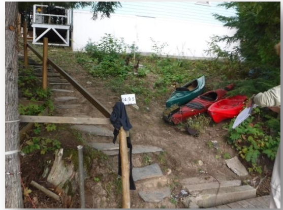
An old walkway requires retrofitting to prevent soil erosion from getting to the lake on Togue Road in Sector 14.
